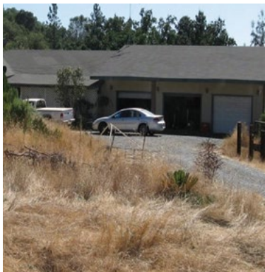
DEFENSIBLE SPACE NONCOMPLIANT
